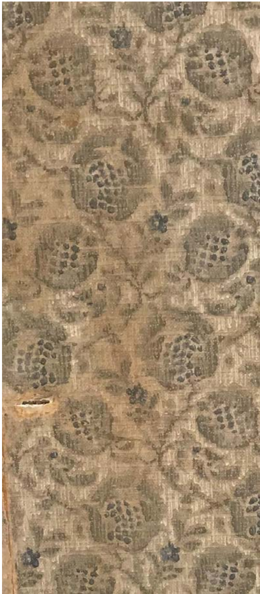
Remnants of original floral printed wallpaper were partly painted over during renovation works in the mid to late 20th century. (PCA)
