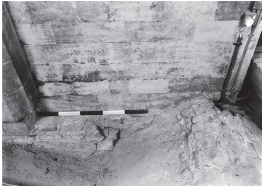
Fig. 43 Masonry at the base of the Bay 5 elevation, showing offset wall and re-use of moulded stones in vaulting (1m scale) ©SCARP
