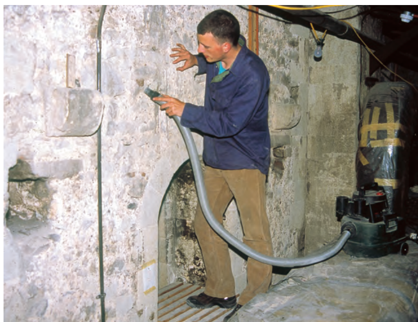
Fig. 6 Cleaning masonry on the north side of the triforium ©SCARP
