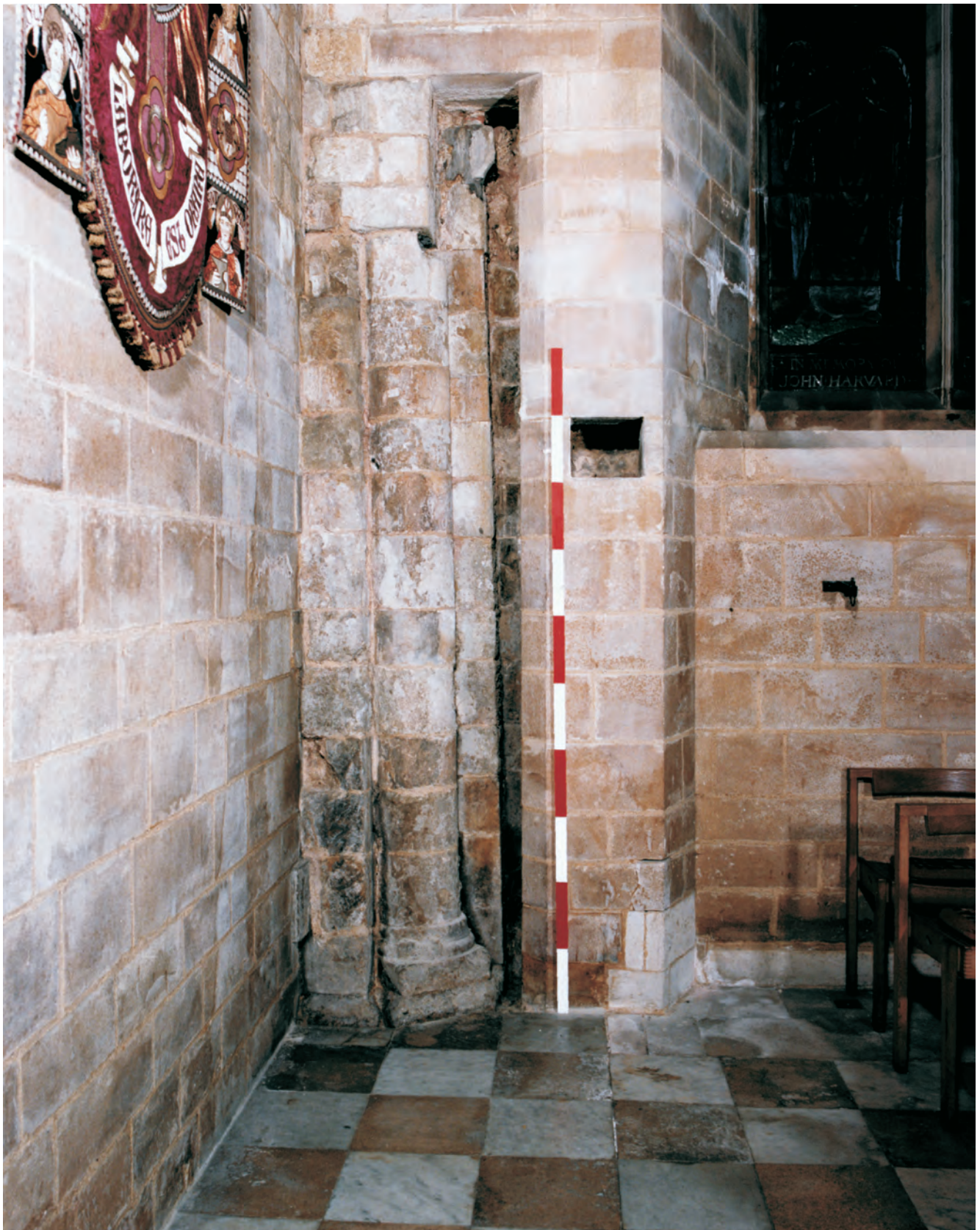
Fig. 49 Nook-shaft in the northeast corner of the northeast transept chapel (2m scale)
