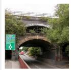
The Lawley Street Viaduct and bridge on Lawley Middleway best shows the original construction of the viaduct with its sandstone dressings and arch with numbered plaque and the brick surfaces of the archway. The later 1893 viaduct can be distinguished by its facing of blue engineering bricks.
