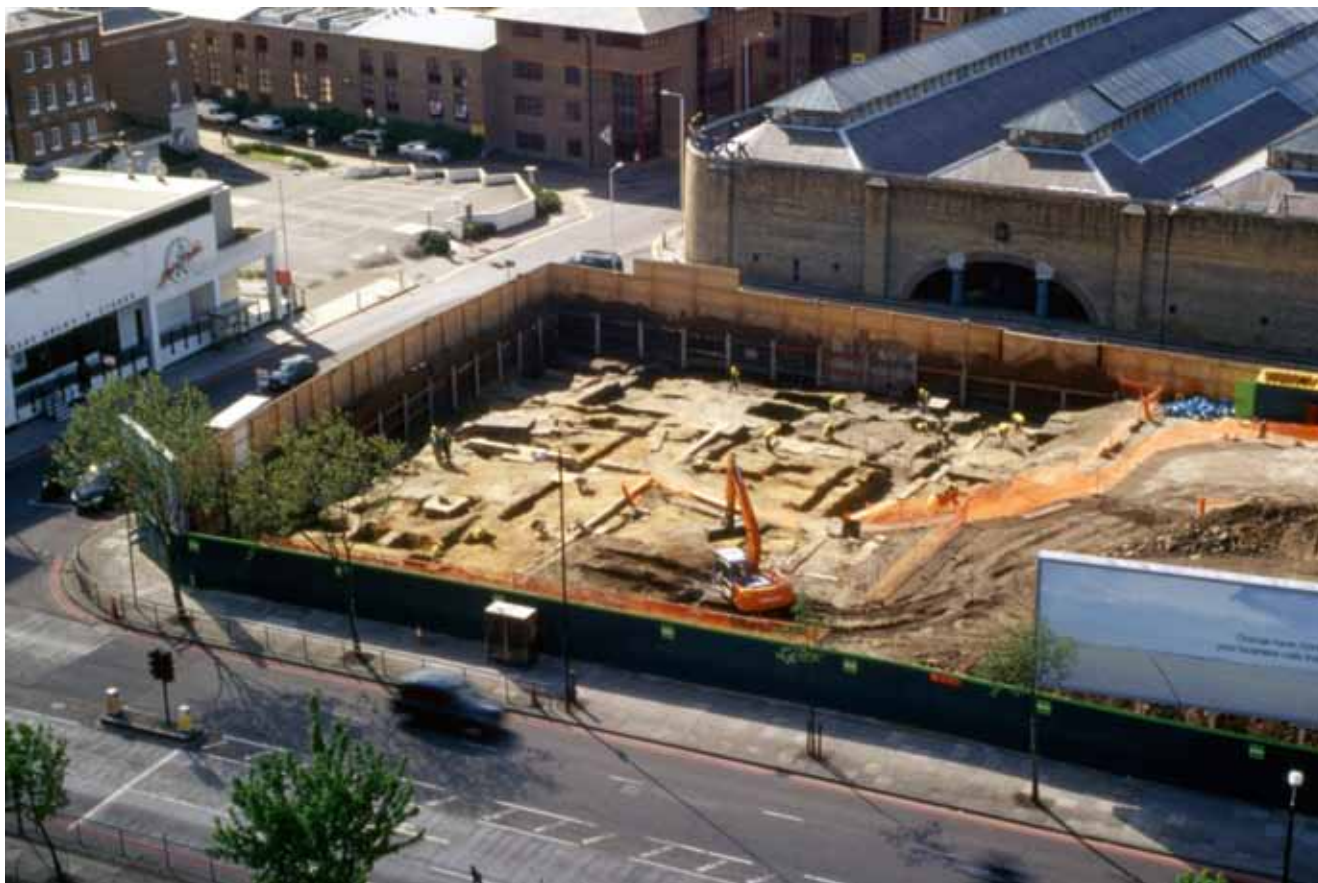
Fig. 3 General view of the Shadwell sites, looking south from the tower of St George in the East, with The Highway running east–west in the foreground and the Tobacco Dock warehouse in the background. Machine ground-reduction is taking place at the Tobacco Dock site in advance of archaeological excavation. To the left is Babe Ruth restaurant, prior to demolition
