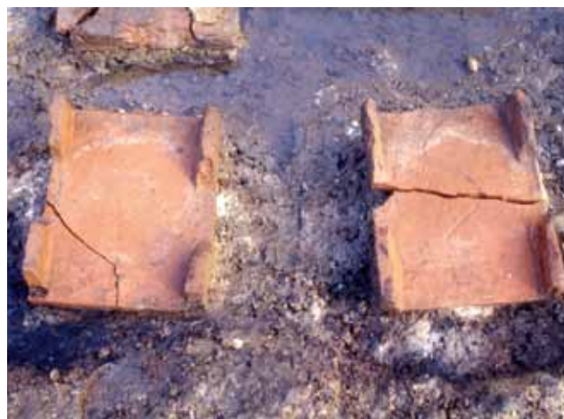
Fig. 42 Close-up of the half-box-flue tiles B[854] and B[855] used in the Room 15 hypocaust pilae stacks
