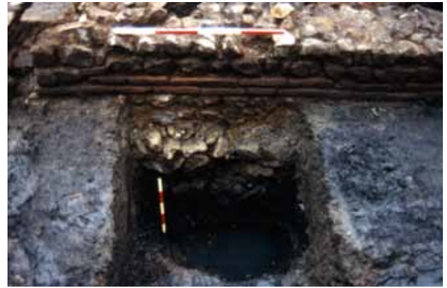
Fig. 13 Part of the foundation level B[1305] for the main south wall of the bath house B[1044]; view looking north; note that the wider Kentish ragstone and chalk foundation supports a superstructure wall of tile facing courses and Kentish ragstone ( opus mixtum ) wall (scales 1m, 0.5m)
